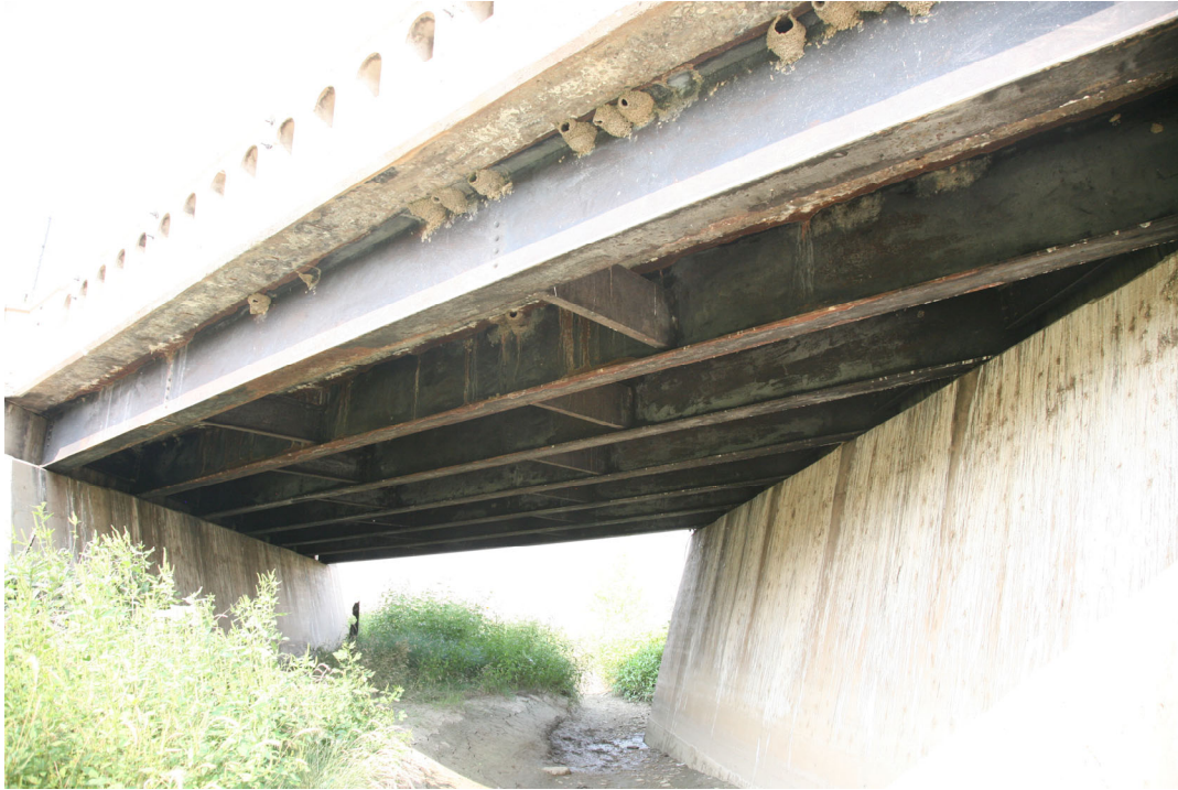
Picture 2 - Pier, Overhang, Deck, Girders
