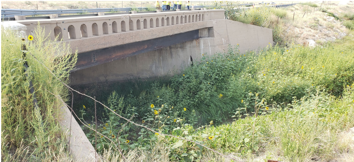
Picture 1 - Bridge M-22-U
